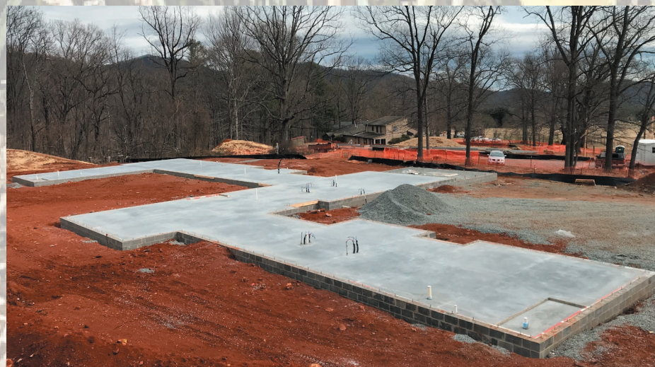
Kenmare is well underway with its finished slab foundation.
